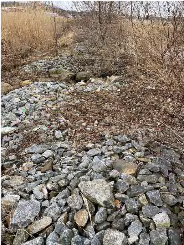
Overflow Weir March 2022 (facing west)
