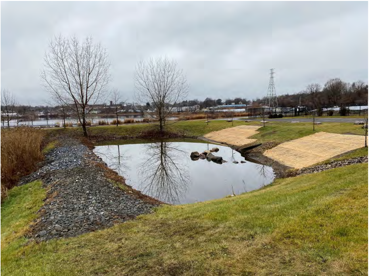
View of restored north forebay December 2022 (facing west)
