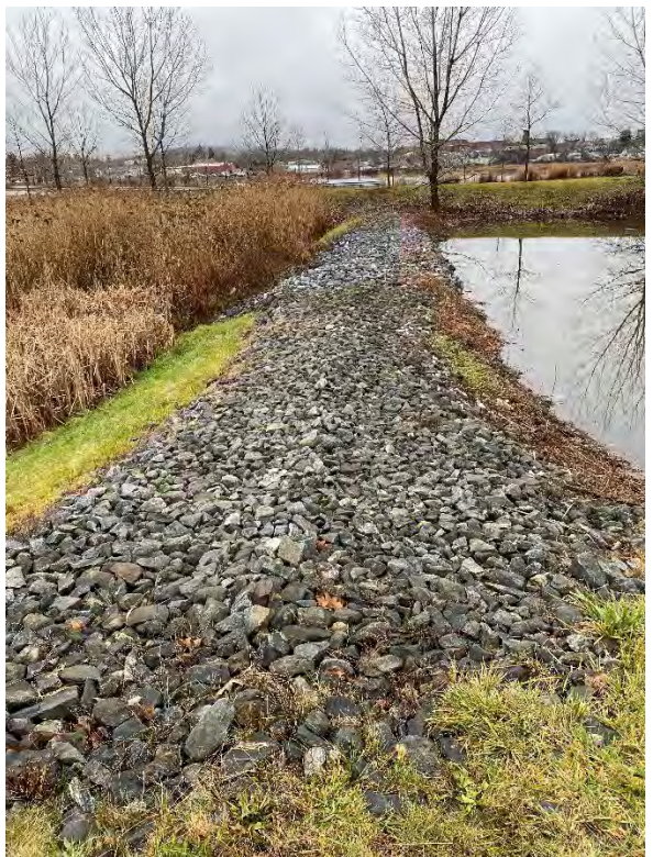
Overflow Weir December 2022 (facing west)
